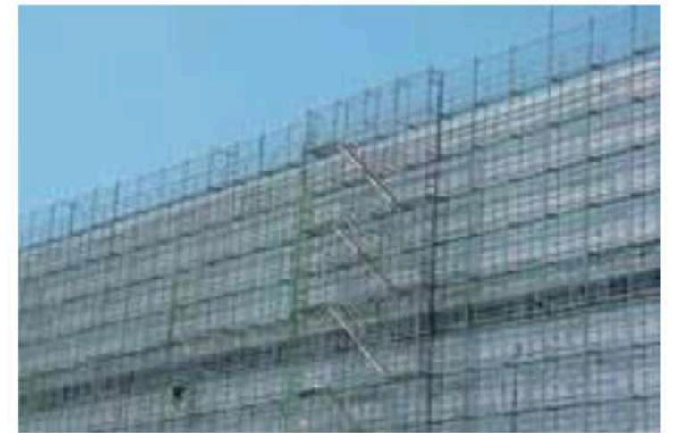
Scaffolding (Restrictions apply)
